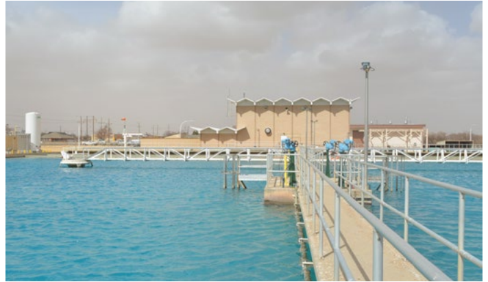
The Osage Water Treatment Plant.
